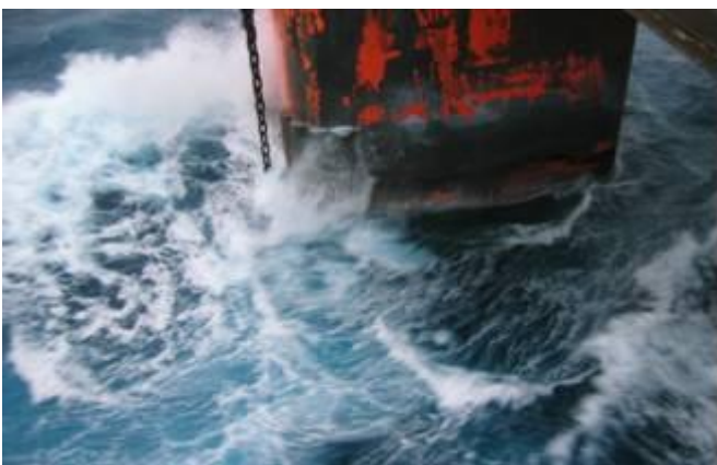
Figure 6.1: Normally there is turbulence in the water around the platform legs. Sea water inlets should be placed where the danger of pollution is at a minimum (Photo: Eyvind Andersen)
