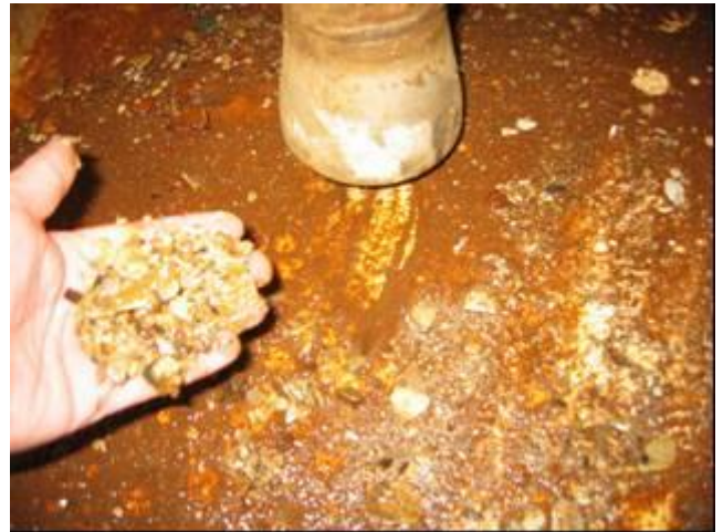
Figure 8.4: During bunkering or in unstable weather particles and sediments in the potable water tanks can be whirled up and sucked into the distribution system, reducing the effect of the UV-radiation. (Photo: Bjørn Løfsgaard)
