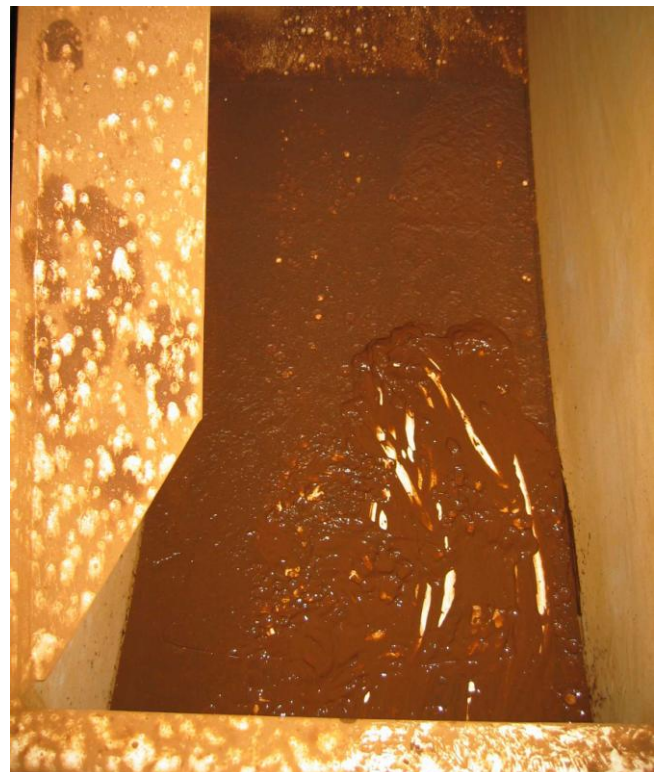
Figure 3.1: Demand for cleaning of tanks at least once a year is set to avoid situations illustrated in the picture above, where there is a layer of mud at the bottom of the tank. Such occurrences have to be handled as a non-conformity case. (Photo: Bjørn Løfsgaard)
