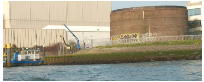
Figure 7.2: This supply base has a water tank that fills up slowly, whilst still providing rapid filling for supply vessels. This way a flushing effect for the water mains is avoided, resulting in cleaner water (Photo: Eyvind Andersen)
