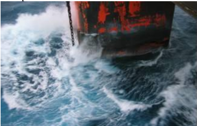
Figure 6.2: Normally there is turbulence in the water around the platform legs. Seawater inlets should be placed where the danger of pollution is minimal (Photo: Eyvind Andersen)
