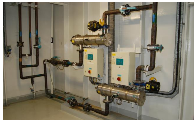
Figure 8.5: This UV unit has two radiation chambers, each with a control panel (white) and an UV sensor (on the front). The black valve closes if the radiation falls below the alarm level. (Photo: Eyvind Andersen)
