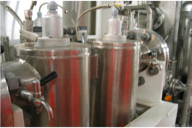
Figure 8.7: UV unit with test taps before and after disinfection (Photo: Eyvind Andersen)
