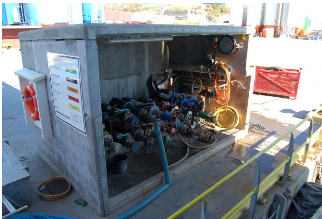
Figure 7.1: Bunkering station on onshore supply base. Water may be polluted prior to entering the supply base, and if supply base routines are weak, both hose connections and hoses may be contaminated (Photo: Eyvind Andersen)
