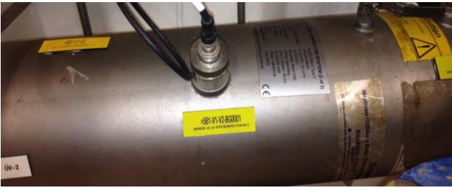
Figure 8.8: Here, the UV sensor is placed on top of the UV chamber (Photo: Eyvind Andersen)
