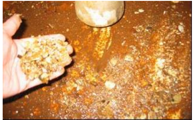
Figure 8.4: During bunkering or in unstable weather, particles and sediments in the potable water tanks can be stirred up and sucked into the distribution system, reducing the effect of the UV radiation. (Photo: Bjørn Løfsgaard)
