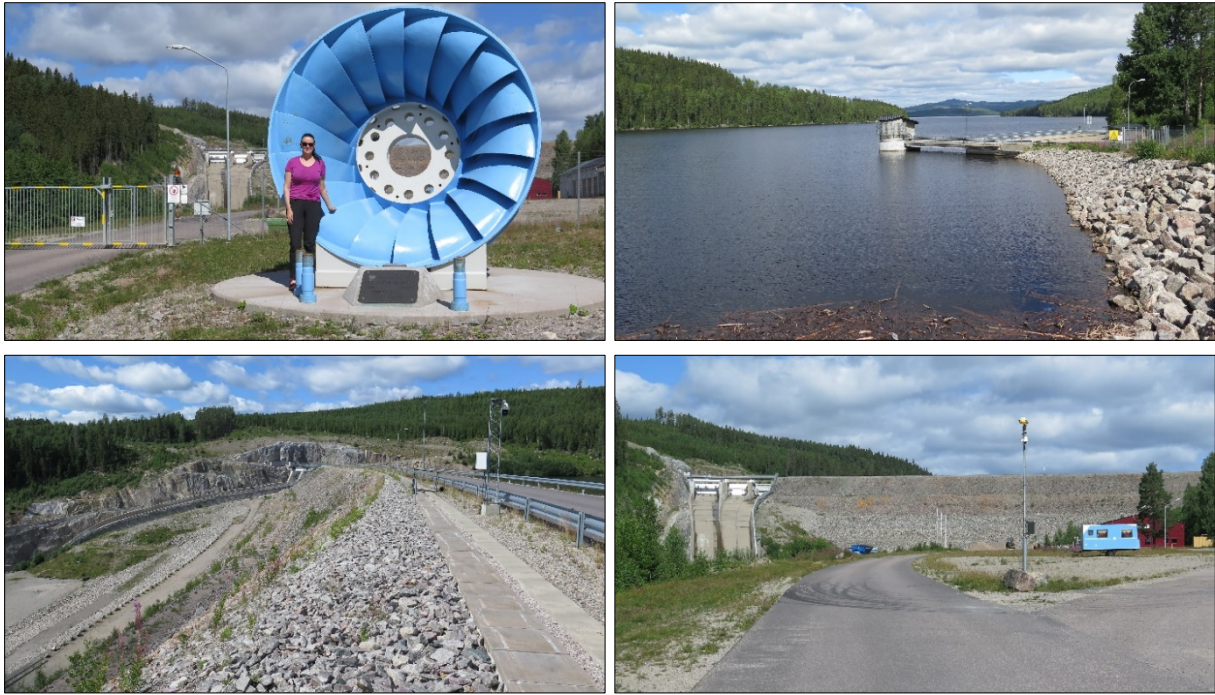
Höljes power station in Sweden including the dam, the old Francis turbine, and the reservoir upstream of the dam. Photos: Eva B. Thorstad.
