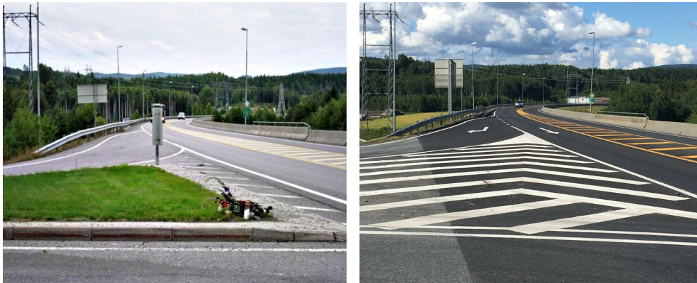
Fig. 9 (Left) The narrow signpost in the middle can hide a motorcycle approaching the intersection over a long stretch (150 m, see Haakenstad, 2015) from the point of view of a driver halting at the entry to the main road. In this photo, a large truck is almost completely covered. This probably happened during a fatal accident at this intersection (Amundsen et al., 2015). Based on the findings of Øhrn et al. (2019), one may speculate that narrow obstructions of view like this signpost are particularly prone to evoking the illusion of absence, and thus a compelling, but potentially misleading conviction that it is safe to enter the main road. (Right) The signpost has later been removed. The photo on the left was taken by Pål Bjerke, Norwegian Public Roads Administration and is reprinted with permission
